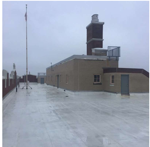
Roof 1 - West View
