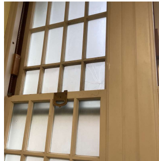
Facade F - Kitchen Locker Room No violations recorded.
