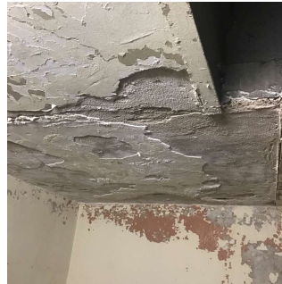
BH2 (Stair 6 and 7)
