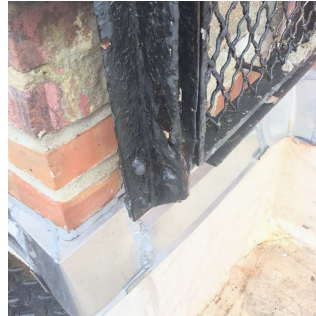
Facade I - East Exit
