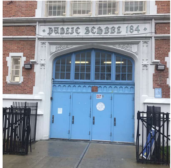
Facade A - Newport Street
