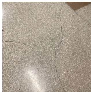
Corridor near Auditorium
