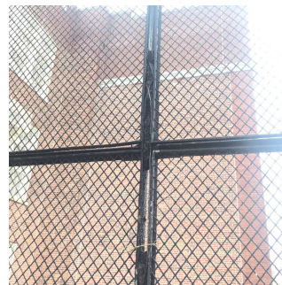
Roof 2 - Facade F
