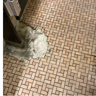
Women Toilet Room - 5th Floor
