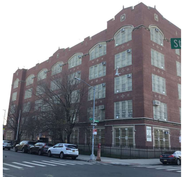
Corner of Riverdale Avenue and Strauss Street - Southeast View
