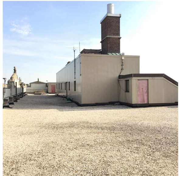
Roof 1 - East View
