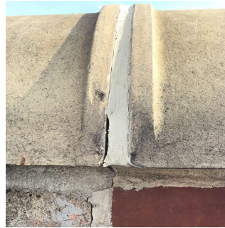
Roof 1 No violations recorded.
