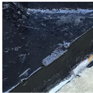
Facade A No violations recorded.
