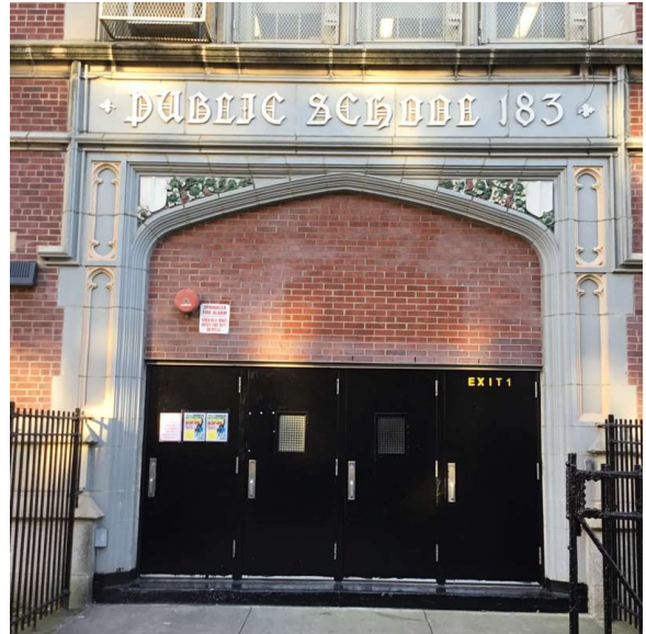
Facade A - Riverdale Avenue
