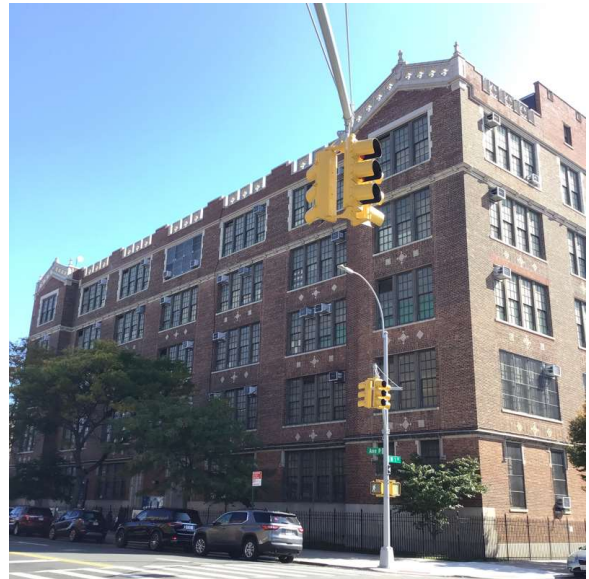
Corner of Dahill Road and Avenue P - Southwest view
