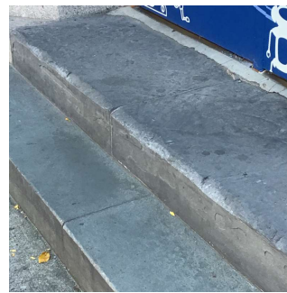
Facade A No violations recorded.
