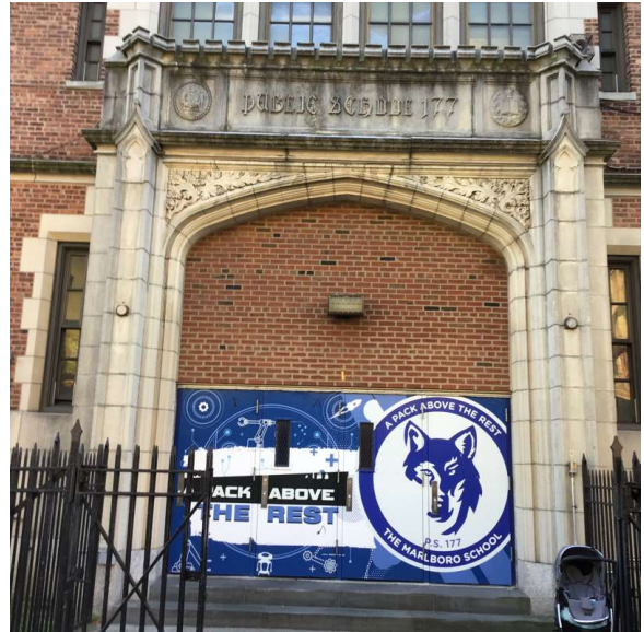
Facade A - Avenue P
