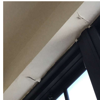
Facade A - Room 309
