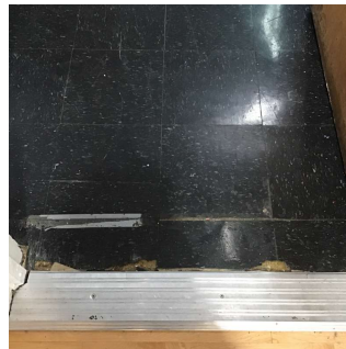
Stair H/1 - Lower Level
