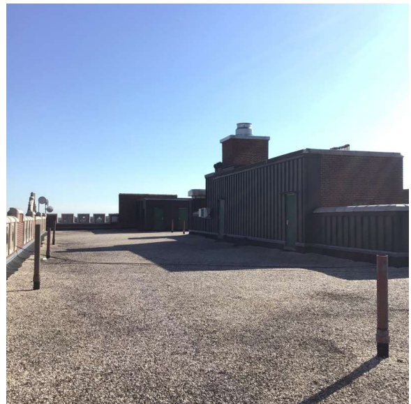
Roof 1 - Southeast view
