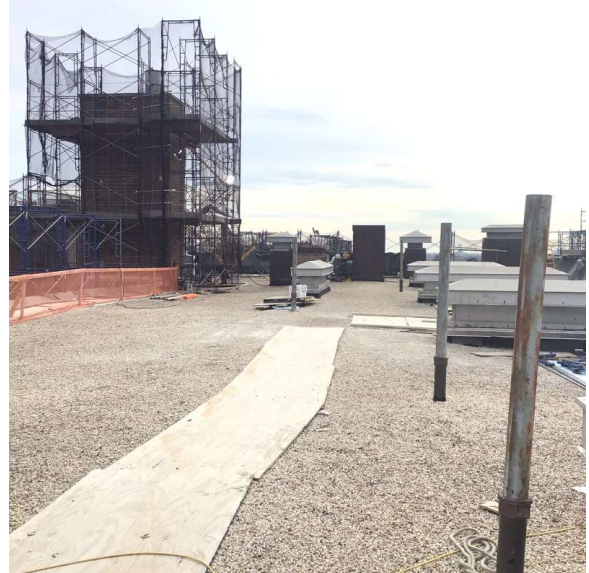
Roof 1 - Southeast View
