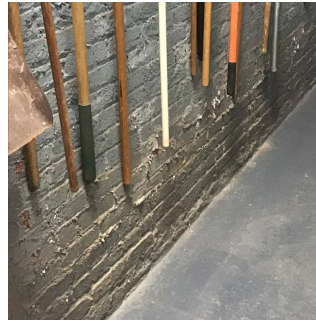
Corridor to Gas Meter Room
