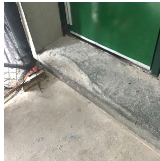
Facade C - Exit 10 Stairs on North corner of the building
