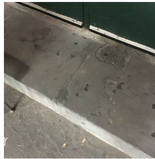
Facade J - Exit 3/4
