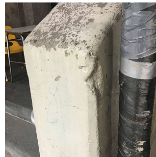
Facade J - Exit 3/4
