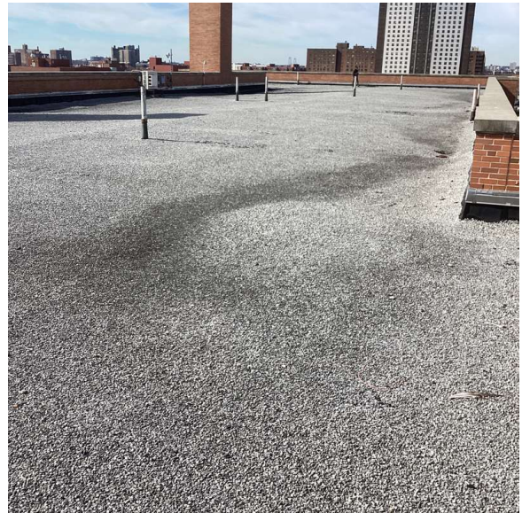
Roof 1 - Southwest View
