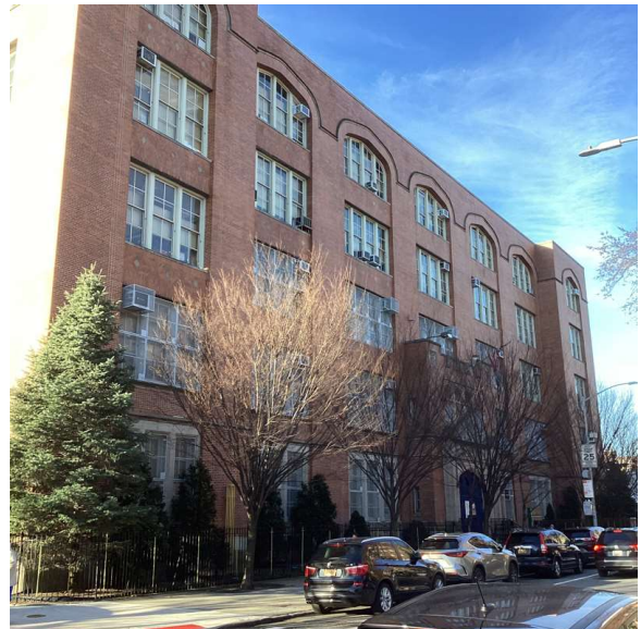
Corner of Dumont Avenue and Alabama Avenue - Southwest View
