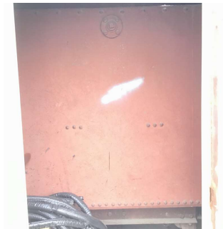
Roof Gravity TANK
