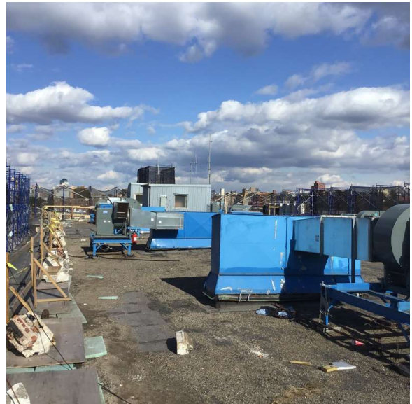
Roof 1 - North View
