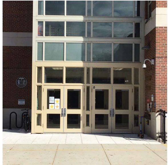
Facade A - 72nd Street
