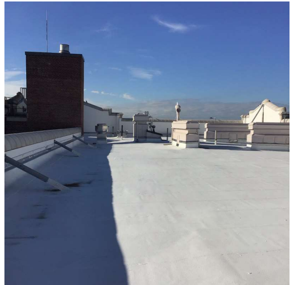
Roof 1 - Southwest View
