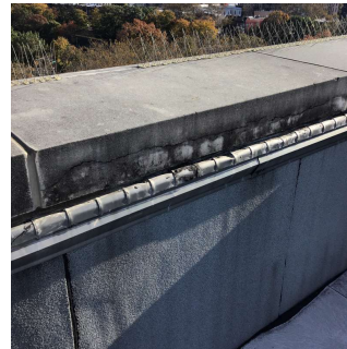
Roof 4 - Facade F
