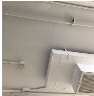
Corridor near Room 206
