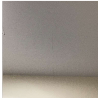
Corridor near Women Toilet - 1st Floor
