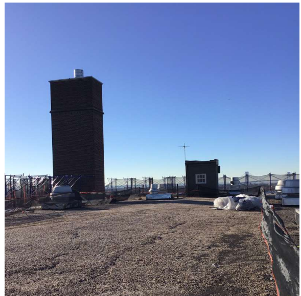
Roof 1 - West View
