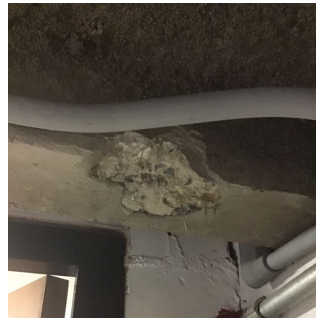
Basement (1937 Addition) - Room 123A
