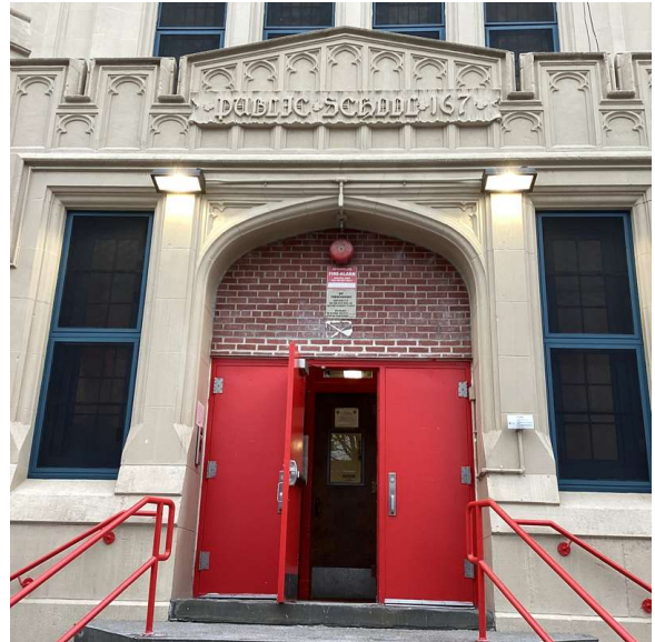
Facade A - Eastern Parkway
