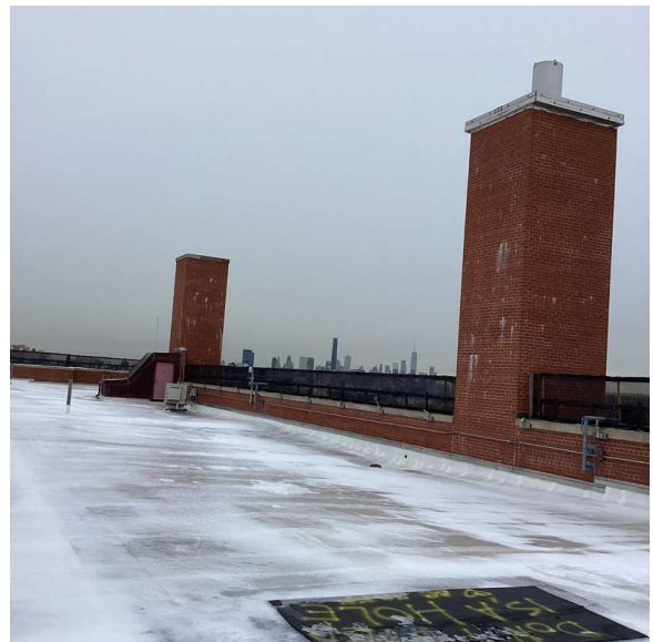
Roof 1 - West View
