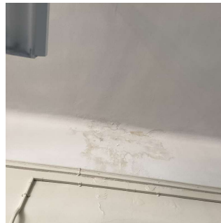
Roof 1 - Room 409 shown, Roof 1 - Rooms 402, 403, 405 , 407 similar
