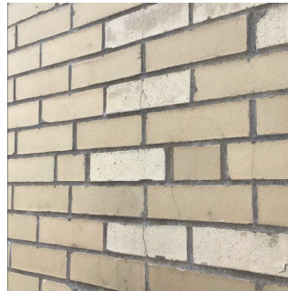
Roof 1 - Chimney 1 No violations recorded.
