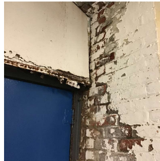
Sub-Basement - Sidewalk Elevator
