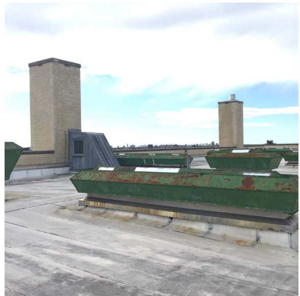
Roof 1 - South view
