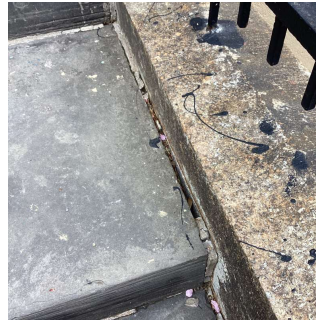
Facade B - Exit 5
