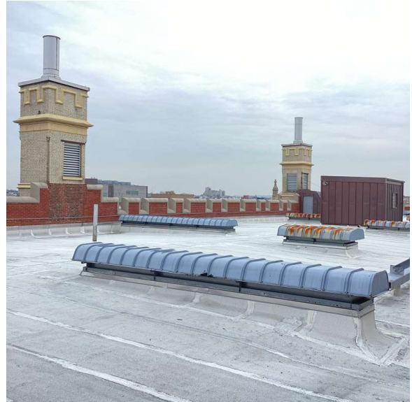
Roof 1 - East View
