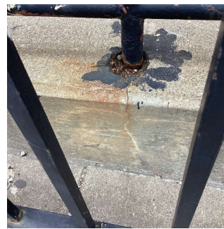
Facade B - Exit 3
