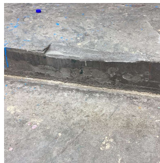
Facade B - Exit 5
