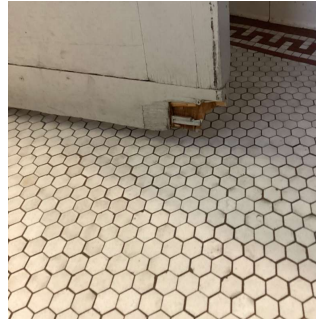
Room 411A No violations recorded.
