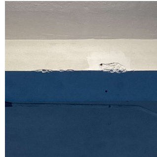
1st Floor - East Multi-Purpose Room No violations recorded.
