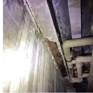
Basement - Mechanical Equipment East No violations recorded.
