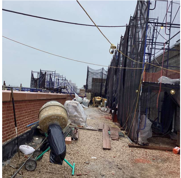
Roof 1 - West View
