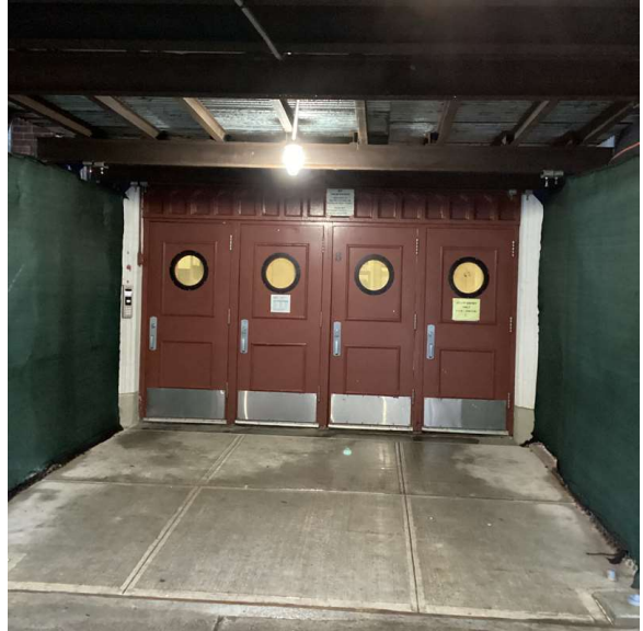
Facade A - Crown Street
