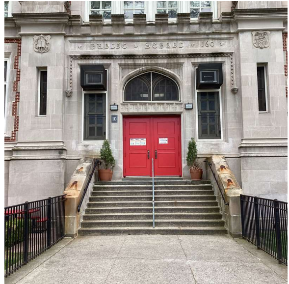
Facade A - Forth Hamilton Parkway
