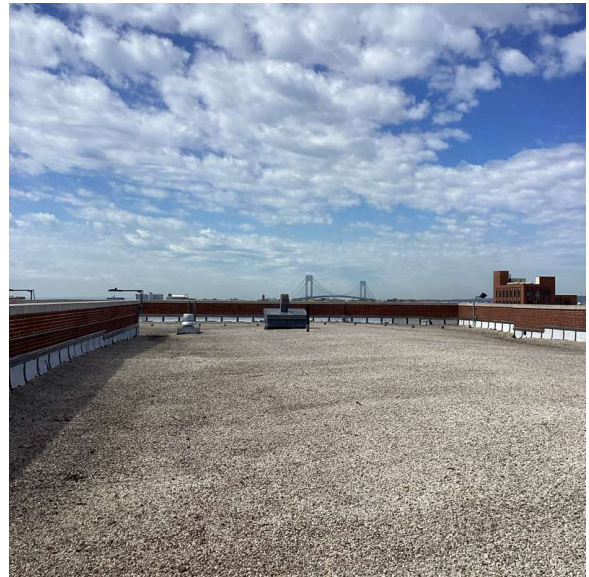
Roof 1 - Southwest View
