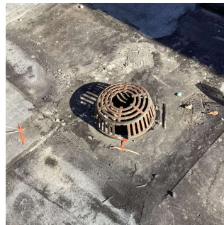
Roof 1 - Above Room 412
