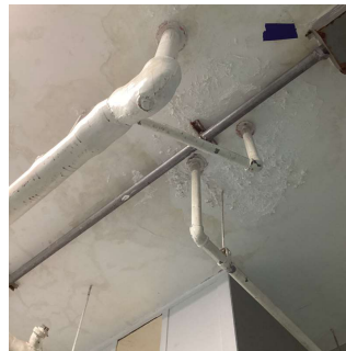
Near Stair A
