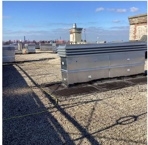
Roof 1 - West View
