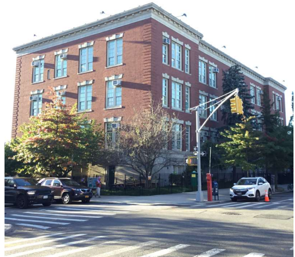
Corner of 11th Avenue and Windsor Place - South View
