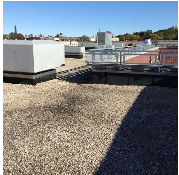
Roof 1 - North View
