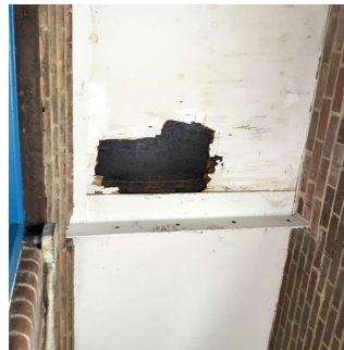
Roof 6 - Exit 6 Vestibule
