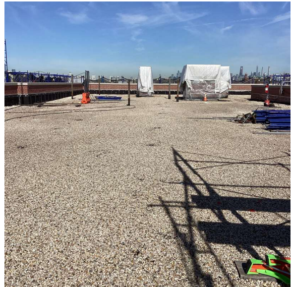
Roof 1 - Northwest View
