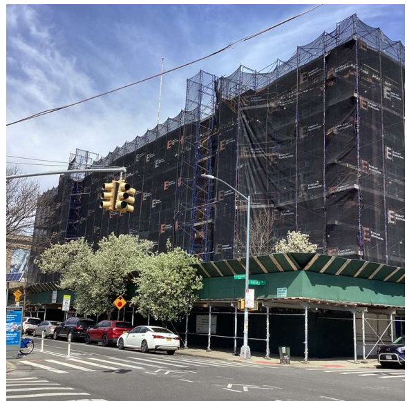
Corner of Halsey Street and Knickerbocker Avenue - North View
