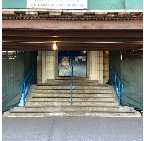
Facade A - Knickerbocker Avenue
