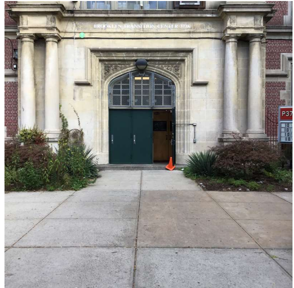
Facade A - Ellery Street
