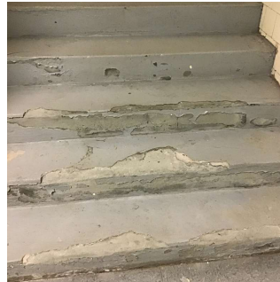
Basement Near Stair C
