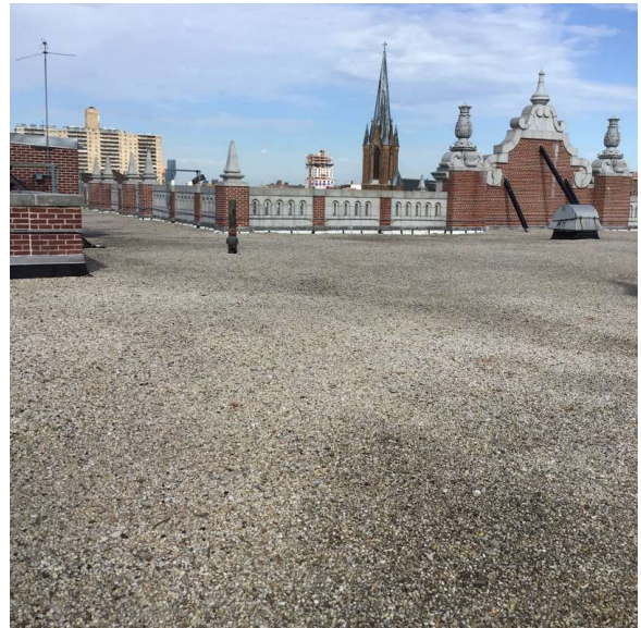
Roof 1 - North View
