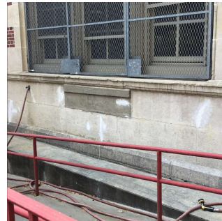
Facade B - Near Ramp
