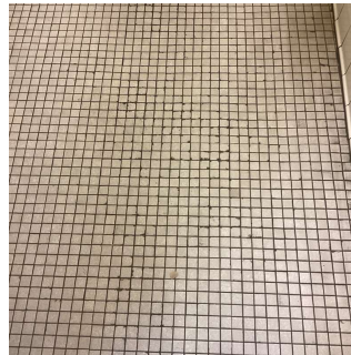
Women Toilet Room - 3rd Floor
