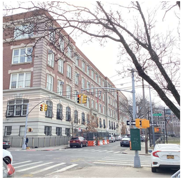
Corner of Noll Street and Central Avenue - South View
