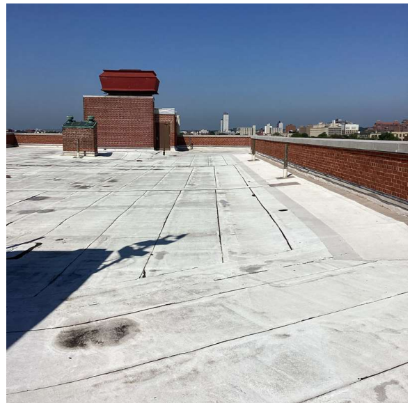
Roof 1 - West View
