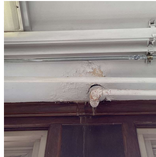
2nd Floor Bridge
