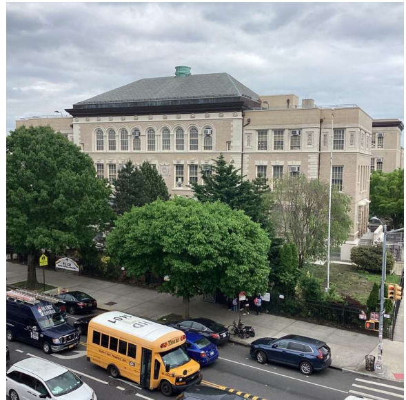
Fort Hamilton Parkway - Southeast View
