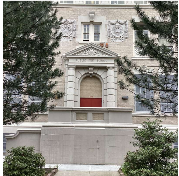
Facade A - Fort Hamilton Parkway
