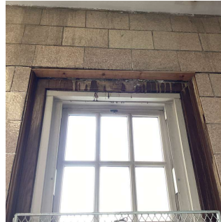
Facade E - 2nd Floor Bridge (Facade K - MDF Room 129, similar)
