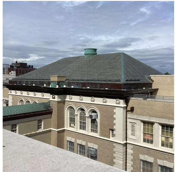
Roof 1 - West View
