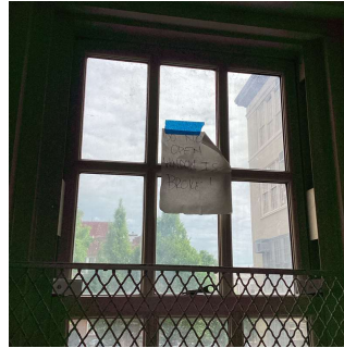
Facade E - 1st Floor Bridge (Facade A - Cafeteria similar)
