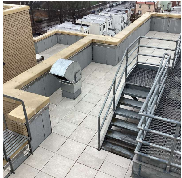
Roof 5 - North View
