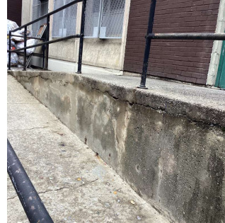
Facade M - Near Exit 11 No violations recorded.
