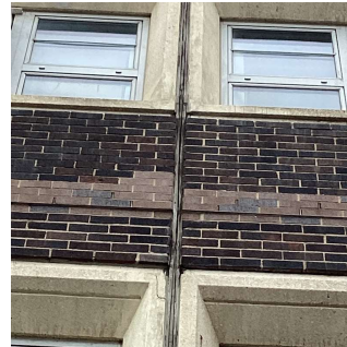
Facade A - Near Main Entrance
