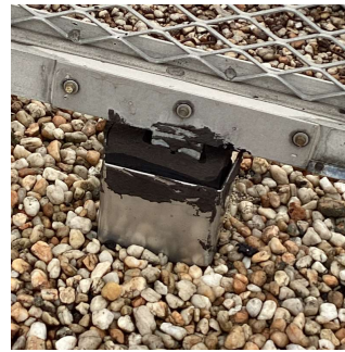
Roof 1 - Near BH2
