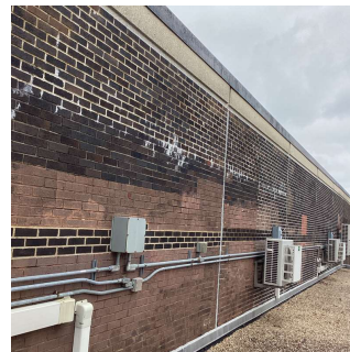
Roof 2 - Near Auditorium Fan Room
