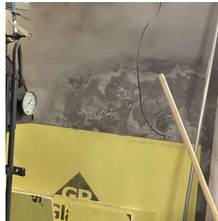
Basement - Boiler Room
