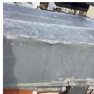
Roof 1 - Facade B
