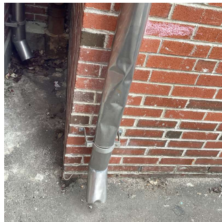
Facade C - Roof 5
