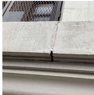
Facade A - Near Main Entrance
