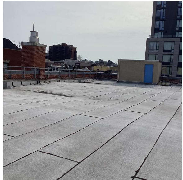
Roof 1 - Southwest View
