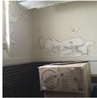
Basement Storage Room near Exit 13
