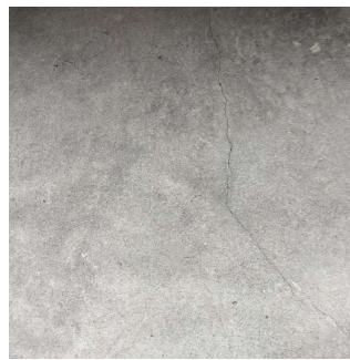
Facade B - Exit 2 and 4 No violations recorded.
