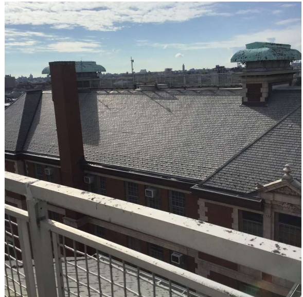
Roof 1 - South View
