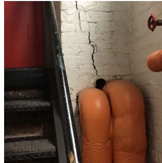
Vault Stair near Stair G
