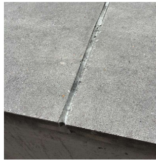
Facade B Exits 2 and 4
