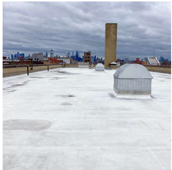
Roof 1 - North View
