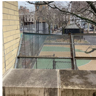
Roof 3 - Facade F
