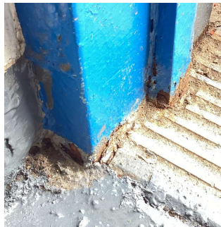
Facade D No violations recorded.
