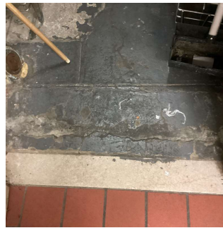
Small Storage Room
