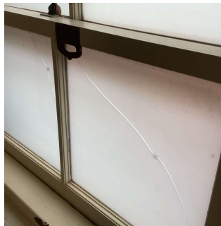
Facade A - Room 109
