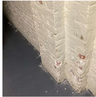
Basement - Stair C
