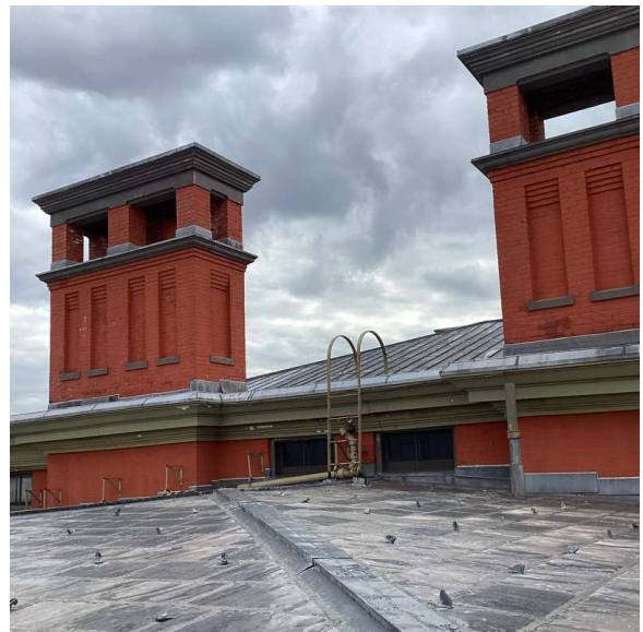
Roof 1 - Northwest View
