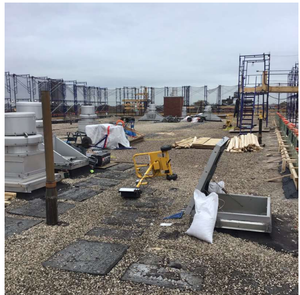
Roof 1 - East View
