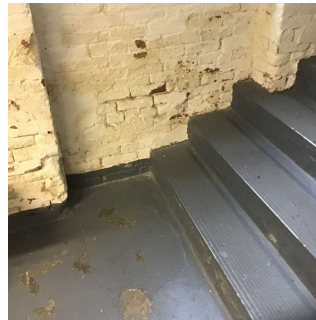
Basement - Exit 7 and 8 Vestibule
