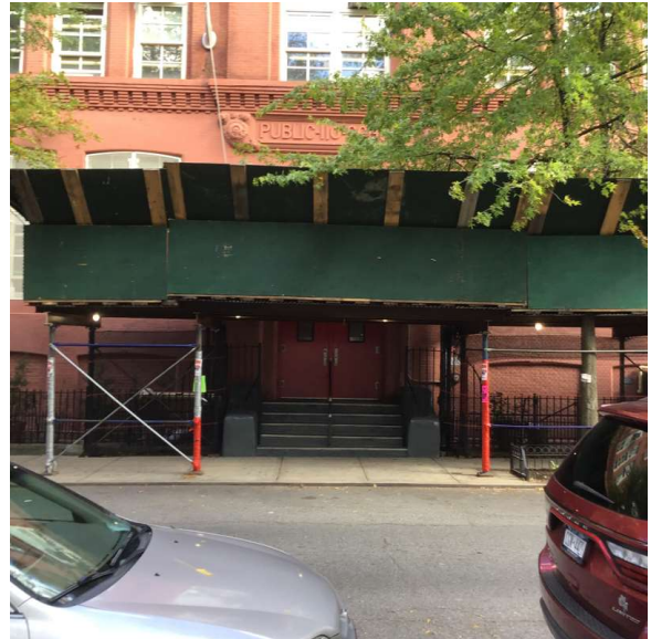
Facade A Monitor Street
