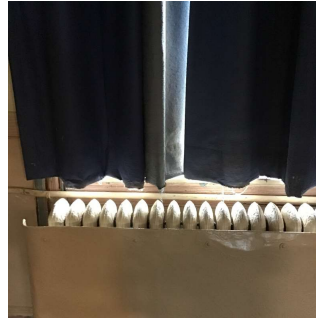
Near Stage No violations recorded.
