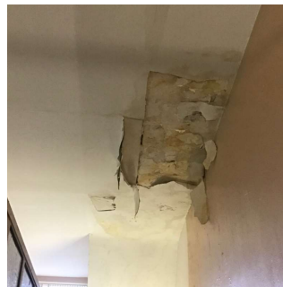
Roof 1 - Stair A4 shown, Roof 5 - 407 similar No violations recorded.
