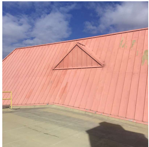
Roof 1 - Northwest View
