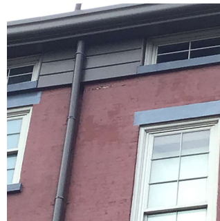
Facade K - North View
