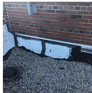
Roof 1 - Facade H No violations recorded.
