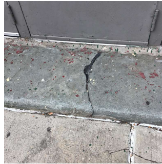
Facade G - Exit 6
