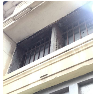
Facade G - Exit 5
