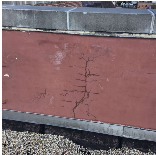
Roof 1 - Facade D 35665478N
