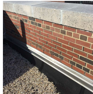
Roof 1 - Facade A No violations recorded.
