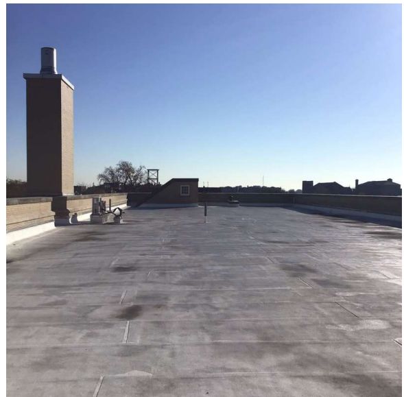
Roof 1 - Southeast View
