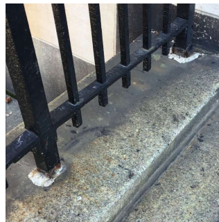
Facade B - Exit 5
