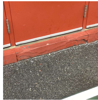
Facade B - Exit 4
