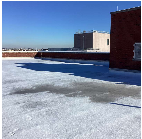
Roof 1 - Northeast View
