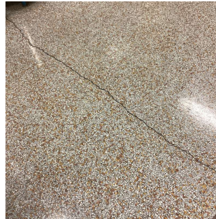
Corridor near room 213
