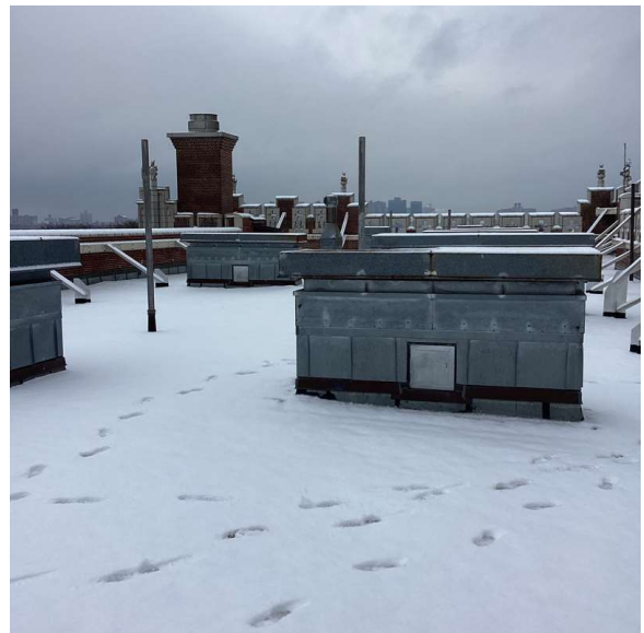
Roof 1 - Southeast View
