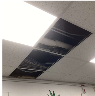
Corridor near Room B26
