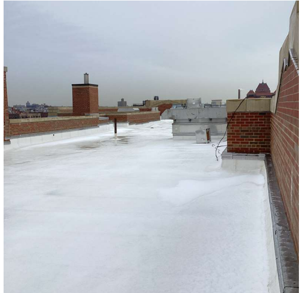
Roof 1 - Southeast View
