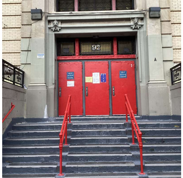
Facade A - Parkside Avenue
