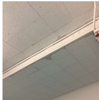
Corridor near Stair F/2
