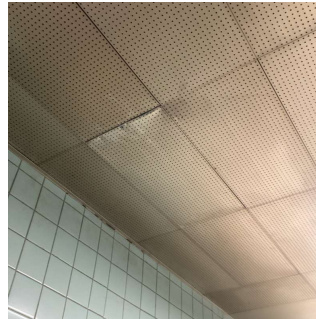
Near Storage Room No violations recorded.
