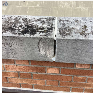
Roof 1 - Facade G
