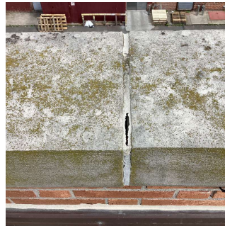
Roof 1 - Facade A
