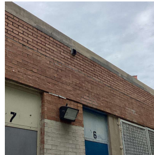
Roof 2 - Facade B
