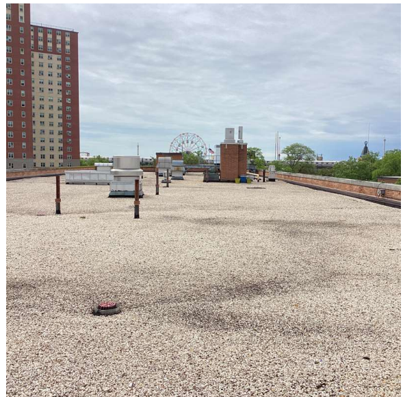
Roof 1 - South View
