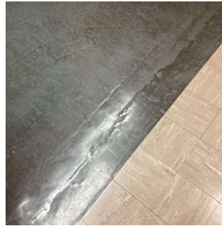
Corridor near Elevator/2
