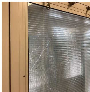
Facade G No violations recorded.
