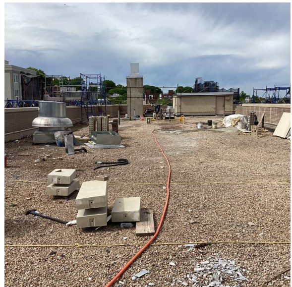
Roof 1 - Southwest View
