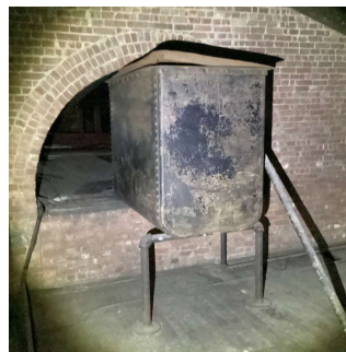
Attic No violations recorded.
