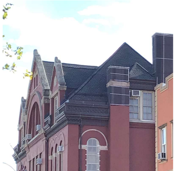
Roof 3 - South View
