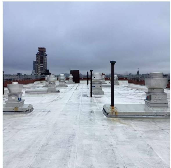
Roof 1 - South View
