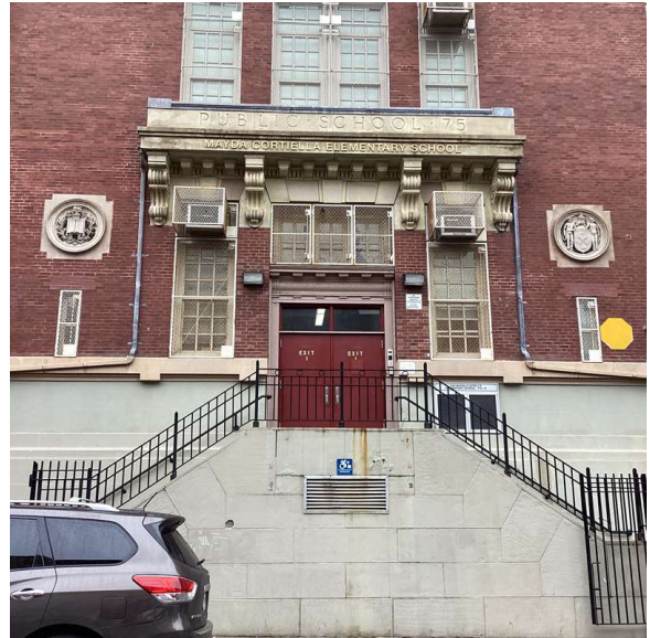
Facade A - Grove Street
