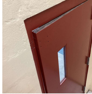
Stair A/B Basement
