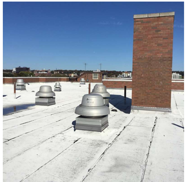
Roof 1 - Northwest View
