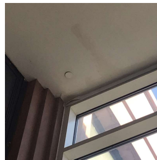
Facade A - 3rd Floor Atrium East Side
