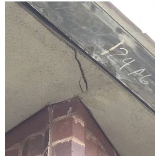
Corner of Facades A and B No violations recorded.
