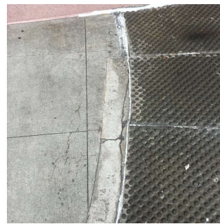
Facade A - Main Entrance No violations recorded.
