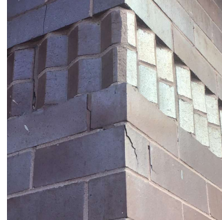
Corner of Facades B and C No violations recorded.
