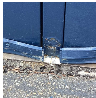
Facade M - Exit 8
