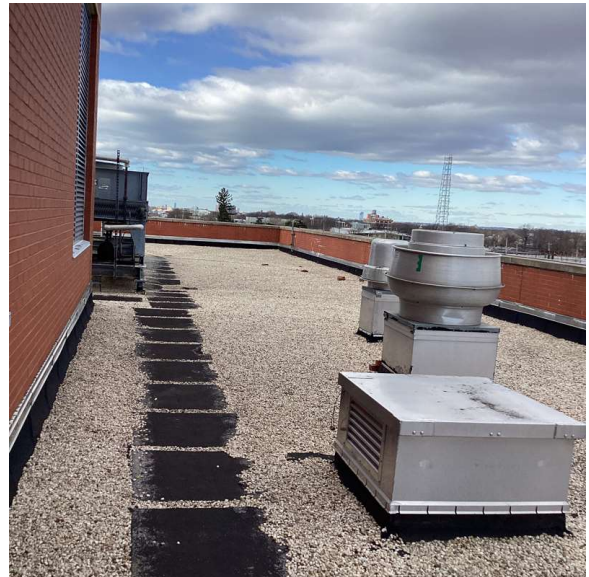
Roof 1 - West View
