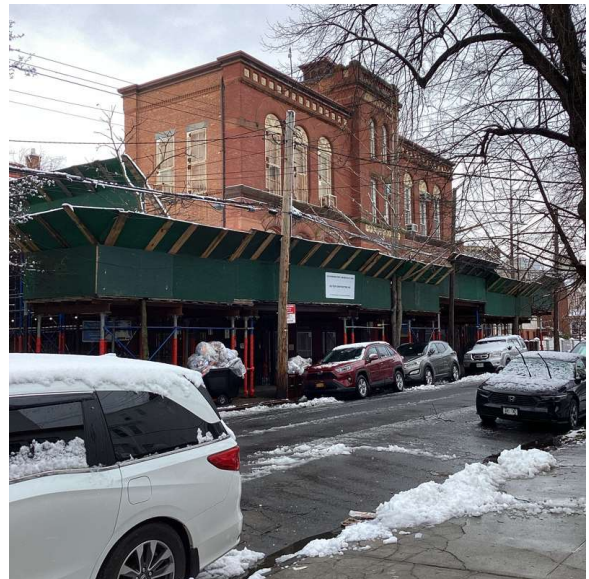
Richmond Street - Northwest View
