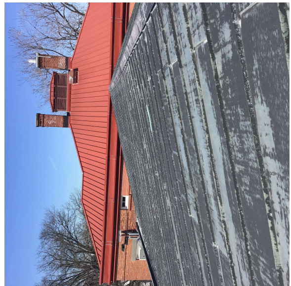
Roof 3 - West View
