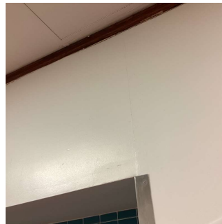
Corridor near Main Office No violations recorded.
