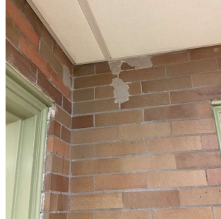
Corridor near room B12 No violations recorded.
