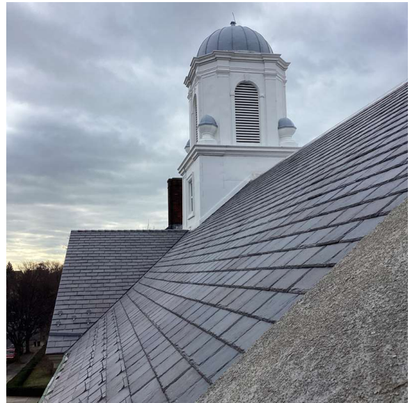
Roof 1 - South View
