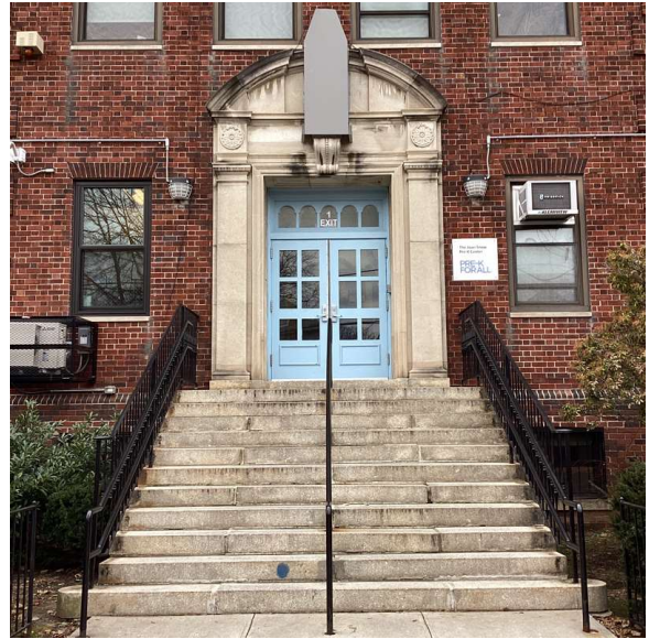
Facade A - East 29th Street
