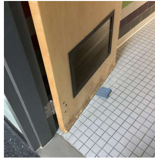
Boys Toilet Room - 3rd Floor
