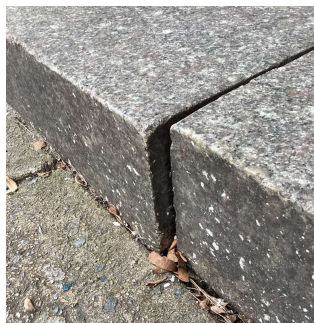
Facade A No violations recorded.
