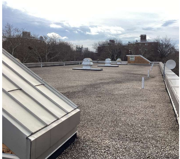
Roof 1 - Southeast View
