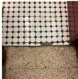
Boys Toilet Room - 1st Floor
