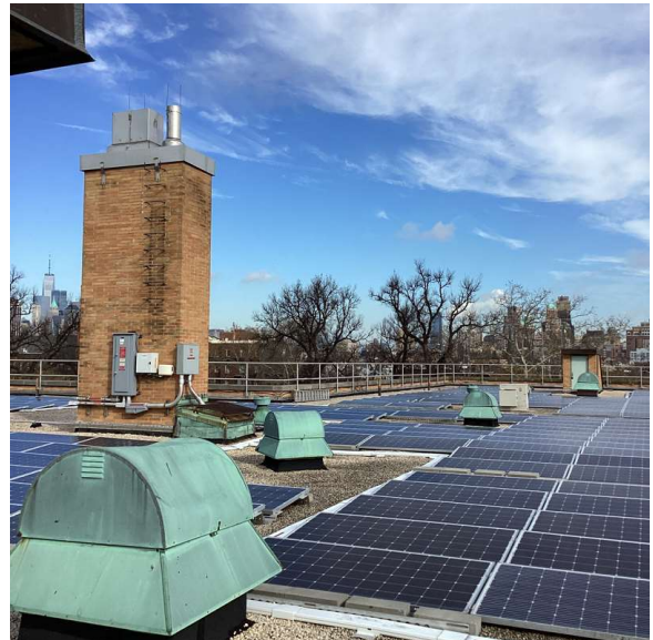
Roof 1 - Northwest View
