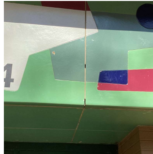
Facade F (Glazed Block)
