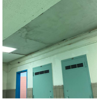
Corridor near Room B11
