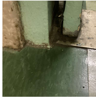
Corridor near Room 207
