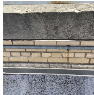
Roof 1 - Facade D
