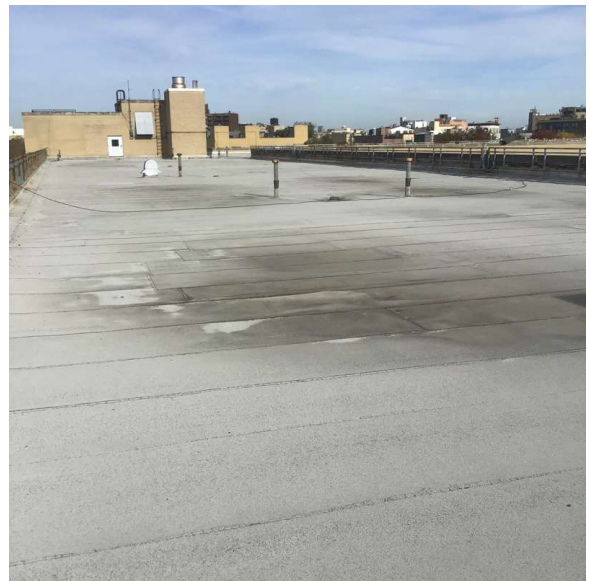
Roof 1 - North View
