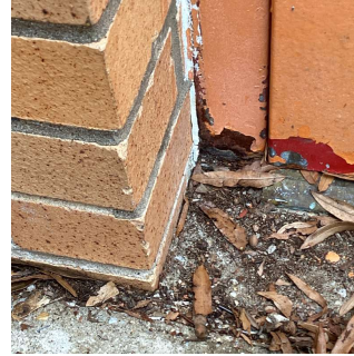
Facade B - Exit 4
