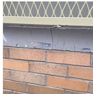
Facade F - Near HC Ramp
