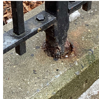
Facade F - Exit 12
