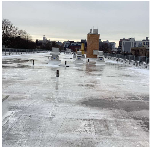
Roof 1 - South View
