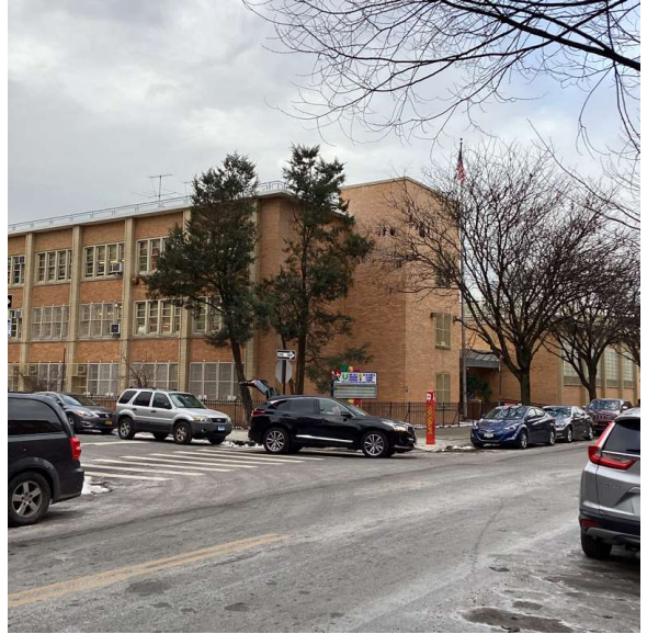
Corner of Irving Place and Gates Avenue - Southwest View
