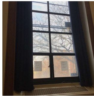
Auditorium Window - similar at Gymnasium
