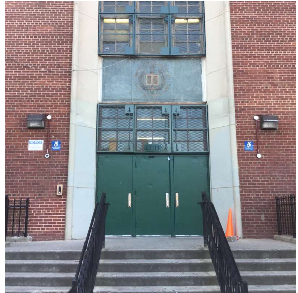
Facade A - 4th Street
